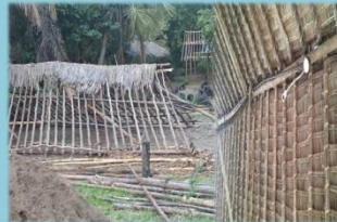
New Eco-Shades & Power Grid installation
