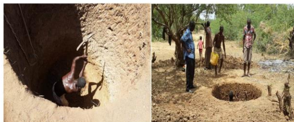
Shallow well digging in progress
