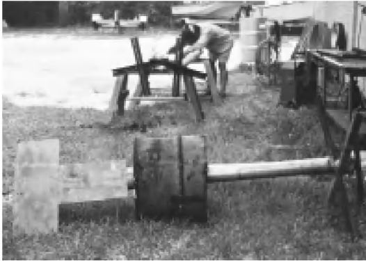
Construction of vandal-proof signs at Boca Grande.
