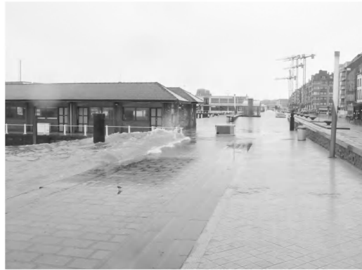
Figure 1: Water reaches quay crest level during a 5-year storm in the harbour of Oostende.
