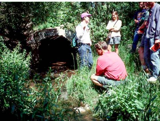
Figure 4 – Strawberry Creek emerges from an underground culvert in Berkeley, California. The creek was exhumed from the pipe in the 1980s, an early and influential example of urban stream “daylighting”. (photo by author, 1992)
