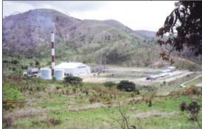
Kanudi Diesel Power Station
