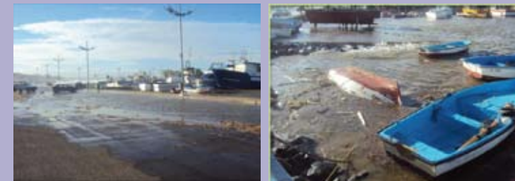
Inundation and damage caused by the 2m rise in sea-level at El Djamilia harbour, 11th September 2010
