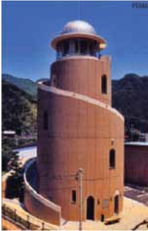
Figure 4.4 Example the Nishiki Tower in the town of Nishiki, Mie Prefecture, Japan
