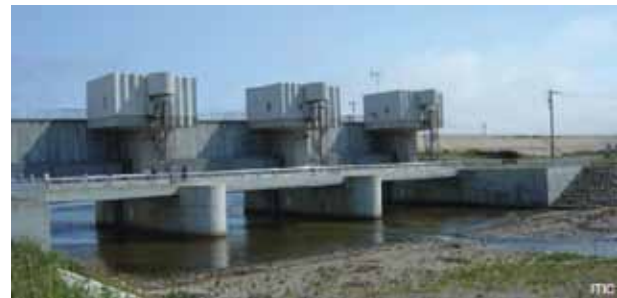
Figure 4.5 Example of water gates from Okushiri Island, Japan.
