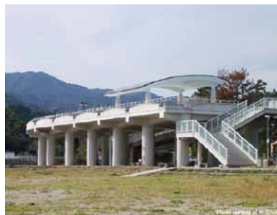
Figure 4.3 Example of an elevated shelter at Shirahama, Tokushima Prefecture, Japan.
