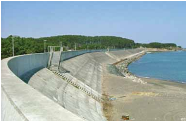
Figure 4.1 Sea wall with stairway evacuation route used to protect a coastal town against tsunami inundation in Japan. Photo courtesy of River Bureau, Ministry of Land, Infrastructure and Transport, Japan.
