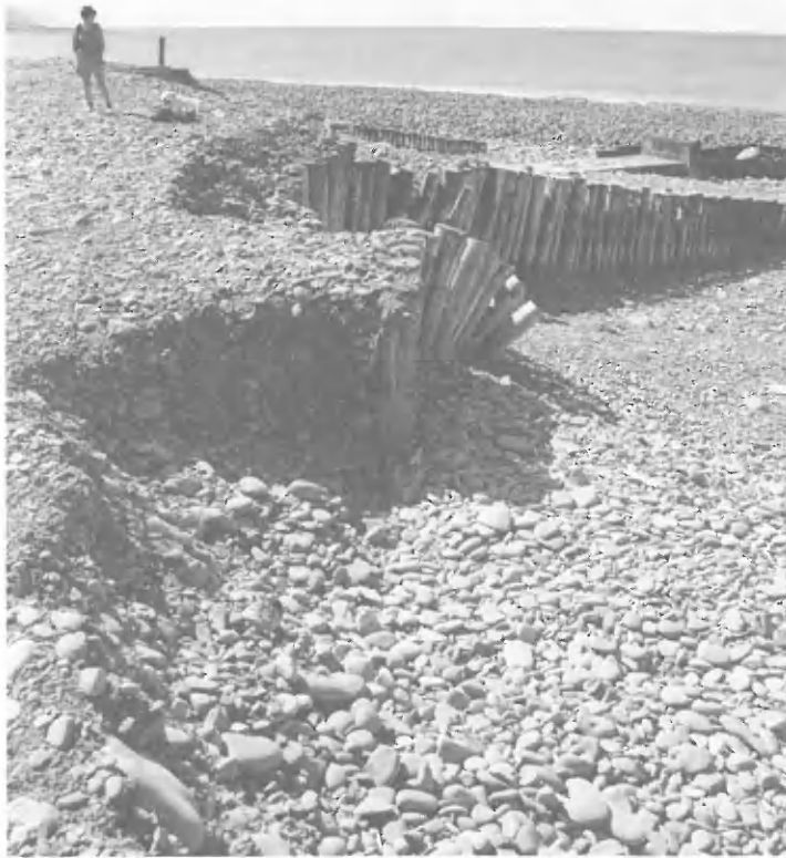
FIG. 1. Groynes east of the New Works outfall ca 1995, looking west. Top. General view. The village is Porlock Weir. Bottom. Detail, showing erosion on the eastern (down-drift) side of the groynes.
