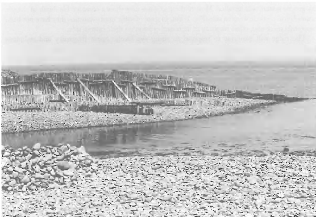
FIG. 5. The 'near terminal' groyne protecting the entrance to the Harbour.
