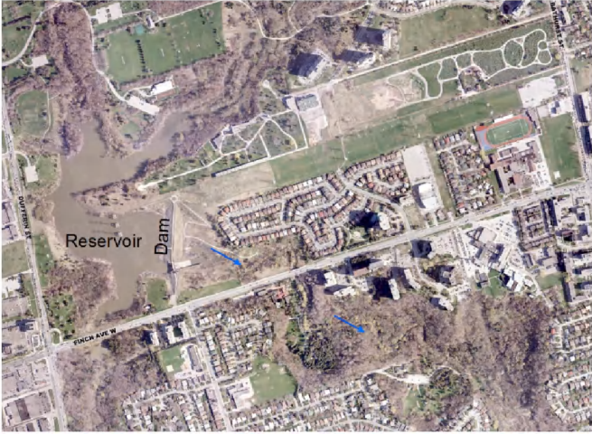
Figure 1. View of the dam and downstream valley for Study Area 1.
