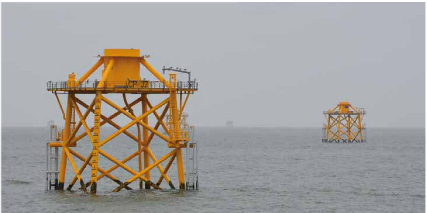
Gulls resting on a jacket foundation during the construction of Phase 2 & 3 of the Thorntonbank wind farm.
