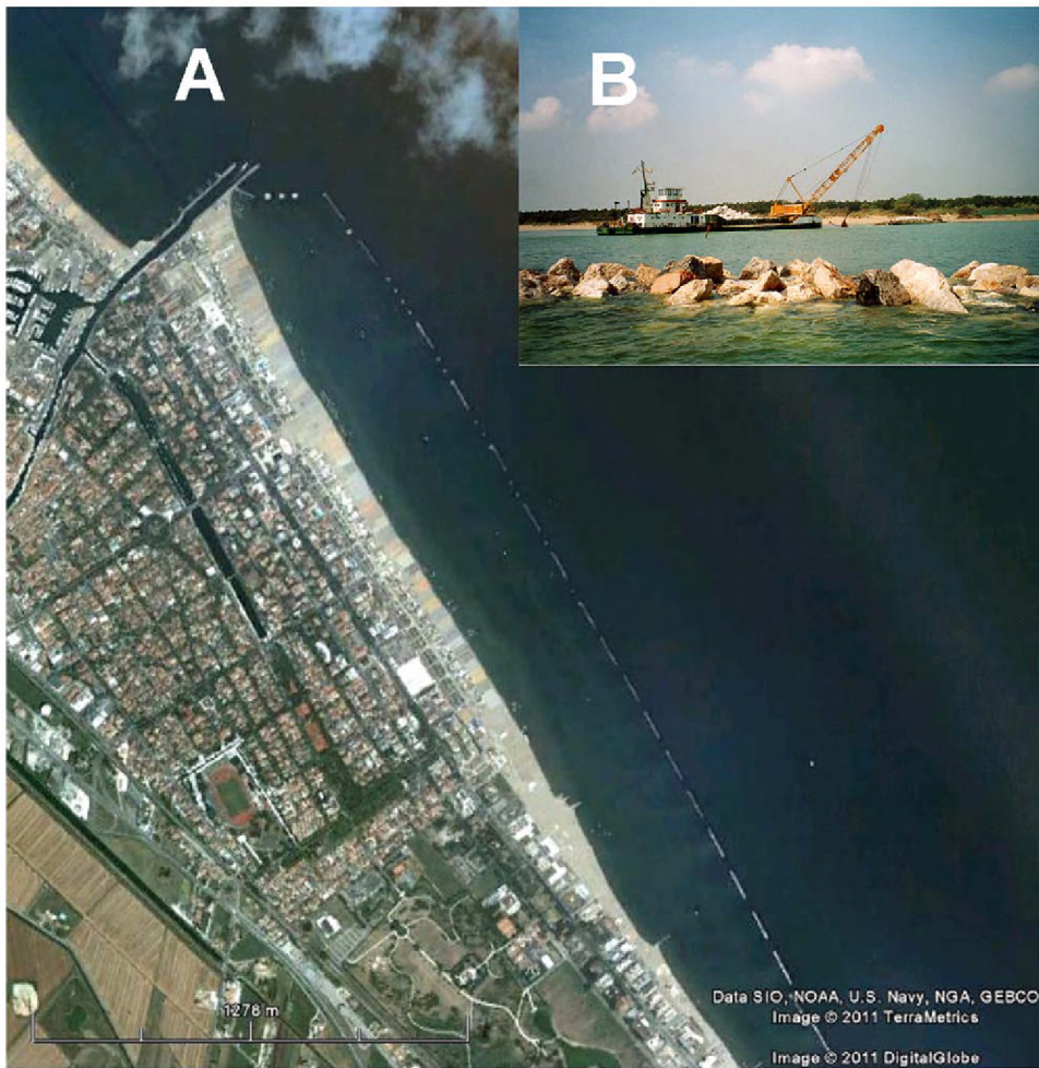
Figure 1. Human-made, coastal defence infrastructures at Cesenatico, along the Italian shores of the north Adriatic sea. A) View of the study area and breakwaters from Google Earth. B) View of a breakwater under maintenance (photo L. Airoidi). doi:10.1371/journal.pone.0022985.g001
