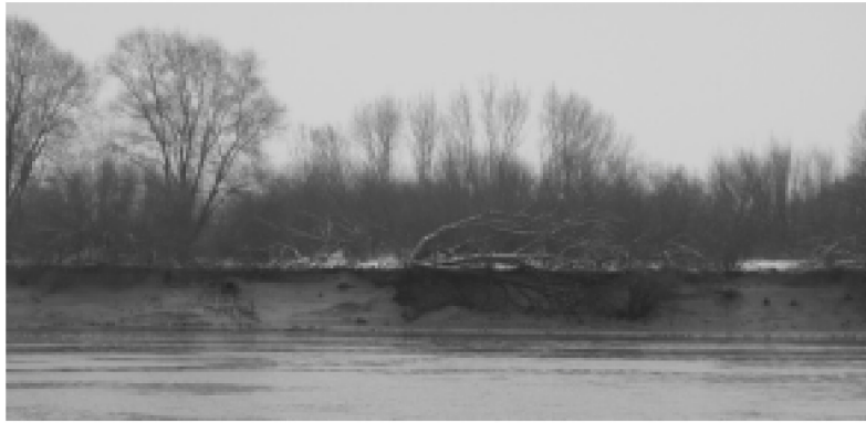
Photo 7.1: Eroded marsh edges in the Schelde estuary.
