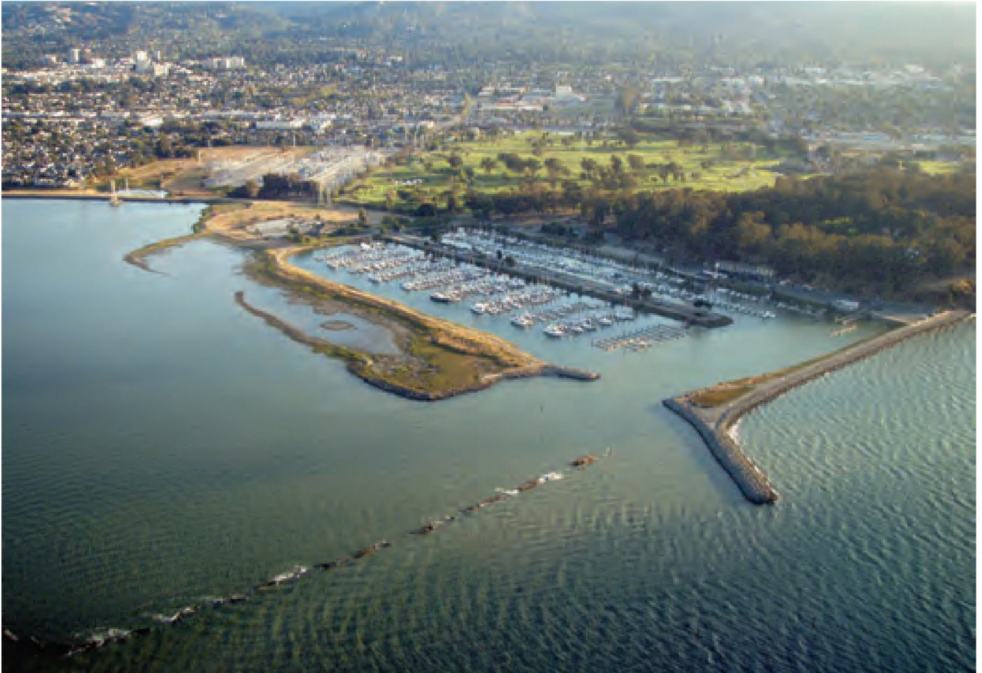
A Marina and Golf Course sit along the San Francisco Bay. The Coyote Point Marina, the Poplar Creek Golf Course and a power substation are just some of the uses for the heavily developed shore along the San Francisco Bay near San Mateo, California. © Gerick Bergsma
