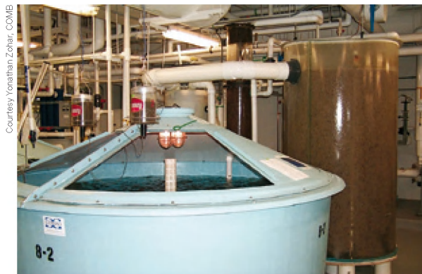
Figure 15. Recirculated fish tank with biofilter (drum on right), which uses beneficial microorganisms to remove chemical wastes from the water
