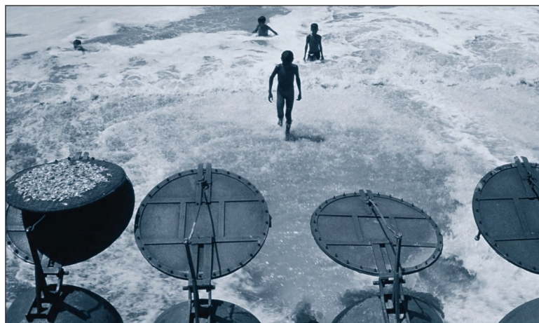
Children swimming near sewage outflow pipes
