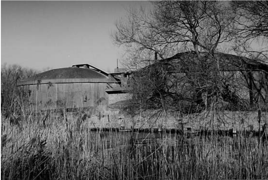
Fig. 7a. A part of the derelict water treatment plant at Groenendijk.
