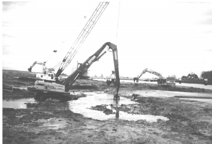
Fig. 5. Phase 2: the 'wet works' or the removal of the jetties and quays of the former Military harbour.
