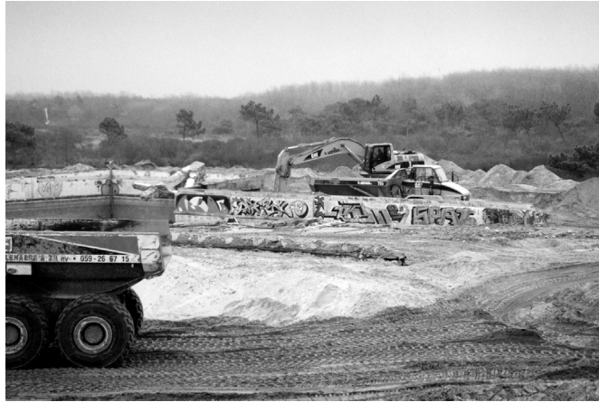
Fig. 6b. The demolition of the Swimming Pool-complex.
