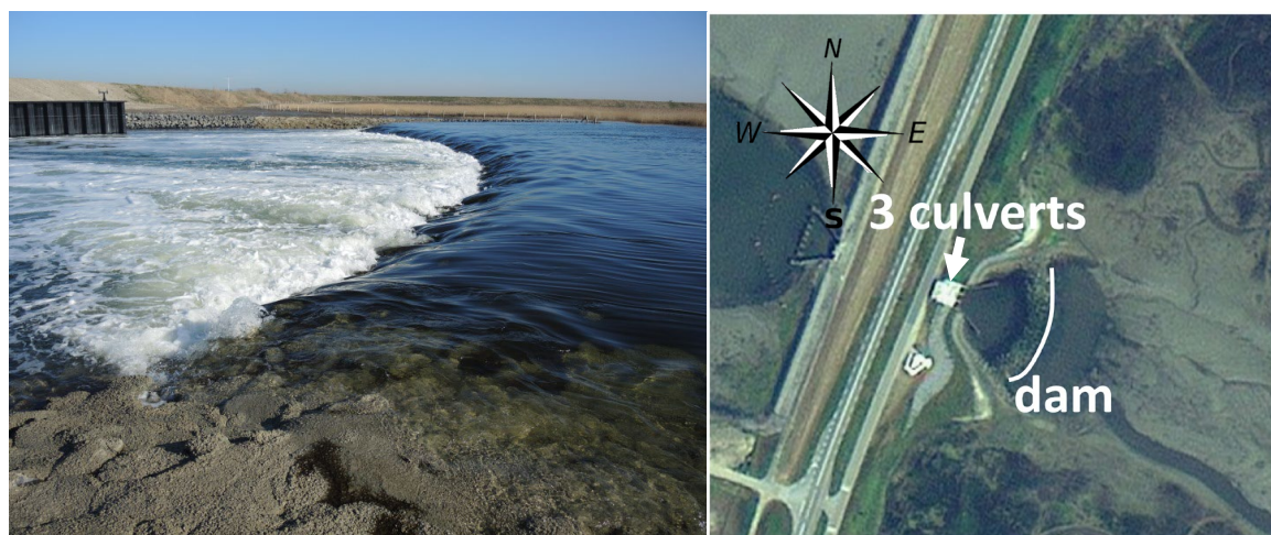
Figure 1-3 Left: Outflow of saltwater during ebb from the Rammegors into the Oosterschelde through the three culverts. Photo: Tom Ysebaert. Right: Position of the dam in the Rammegors area and the three culverts in the inlet.
