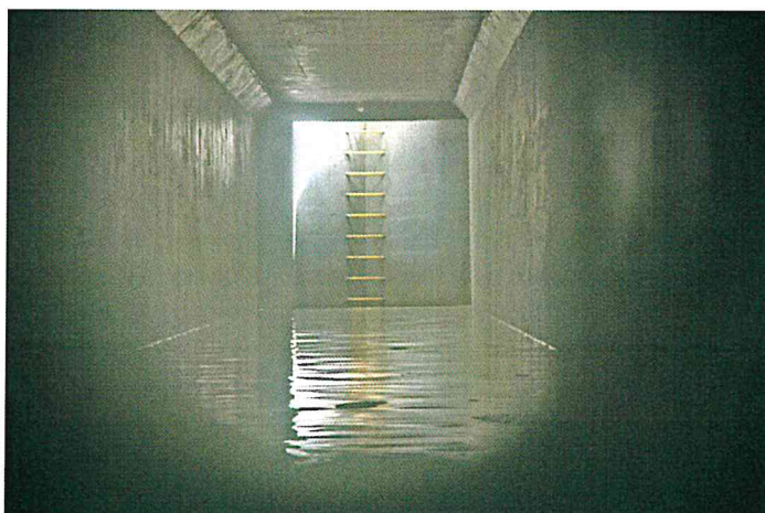
Figure 1: Inside view of one of three subterranean water tanks
