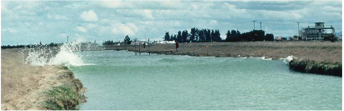
Figure 5.9 | Controlled dambreak hydraulic jump passing along a power canal.
