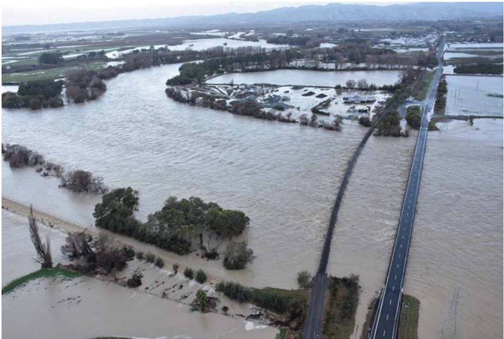
Figure 5.10 | Local flooding (background) outside embankments controlling a major river flood (foreground).
