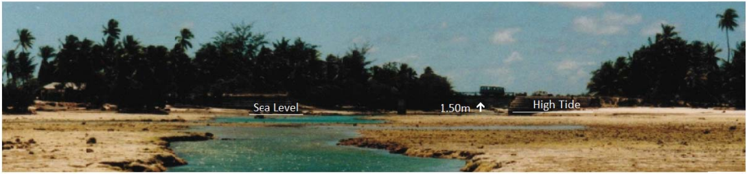
Figure 7.1a | Example of analysis of the selection of design parameters for a coastal bridge at risk from sea level rise.
