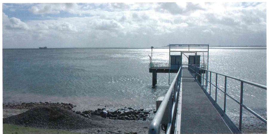
The new jetty provides safe and easy access to the waters of the Marsdiep tidal inlet. Photo: Josje Snoek /NIOZ.
