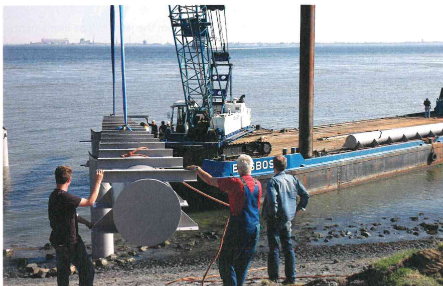
Construction of the gangway of the new jetty.
