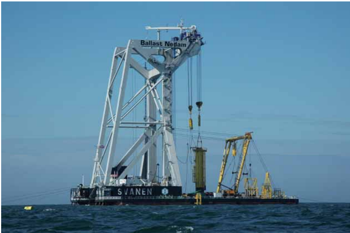
Figure 40. Windfarm (pile driving) construction activities 16 April 2006 (C.J. Camphuysen).
