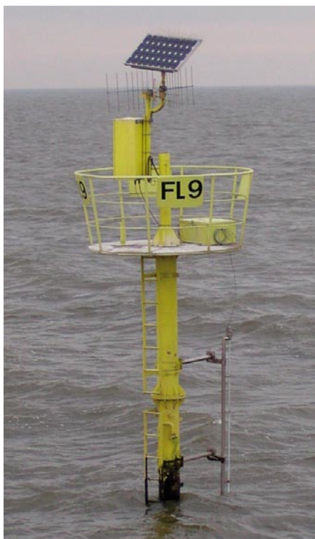
..... Photo 6 FL9-location, view from SE, Jan 2005
