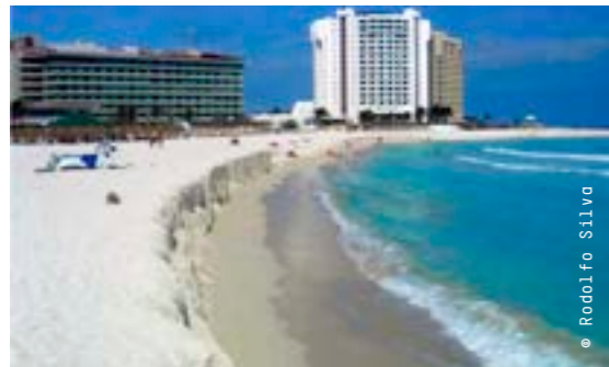
NEW SAND nourishments on Cancun beach start eroding immediately.
