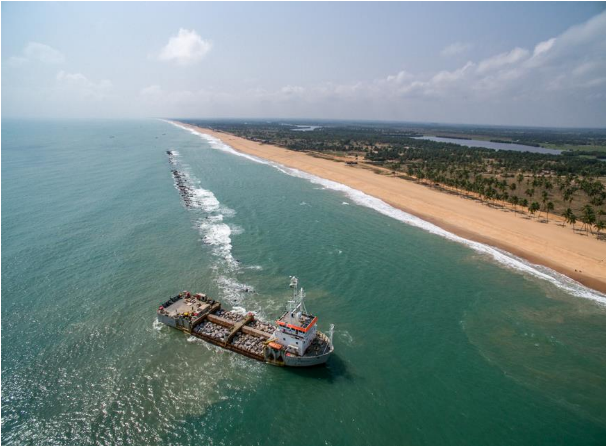
Figure 2-1. Side stone dumping vessel Pompei installing the submerged breakwater
