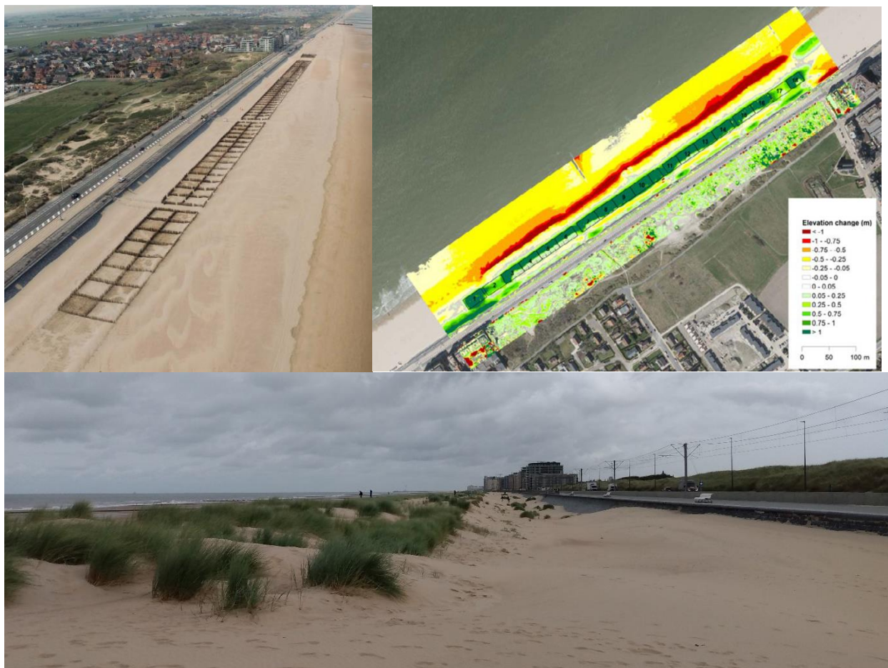
Figure 15 – Living Lab Raversijde (BE) Demonstrator, Dune-in-front-of-Dike
