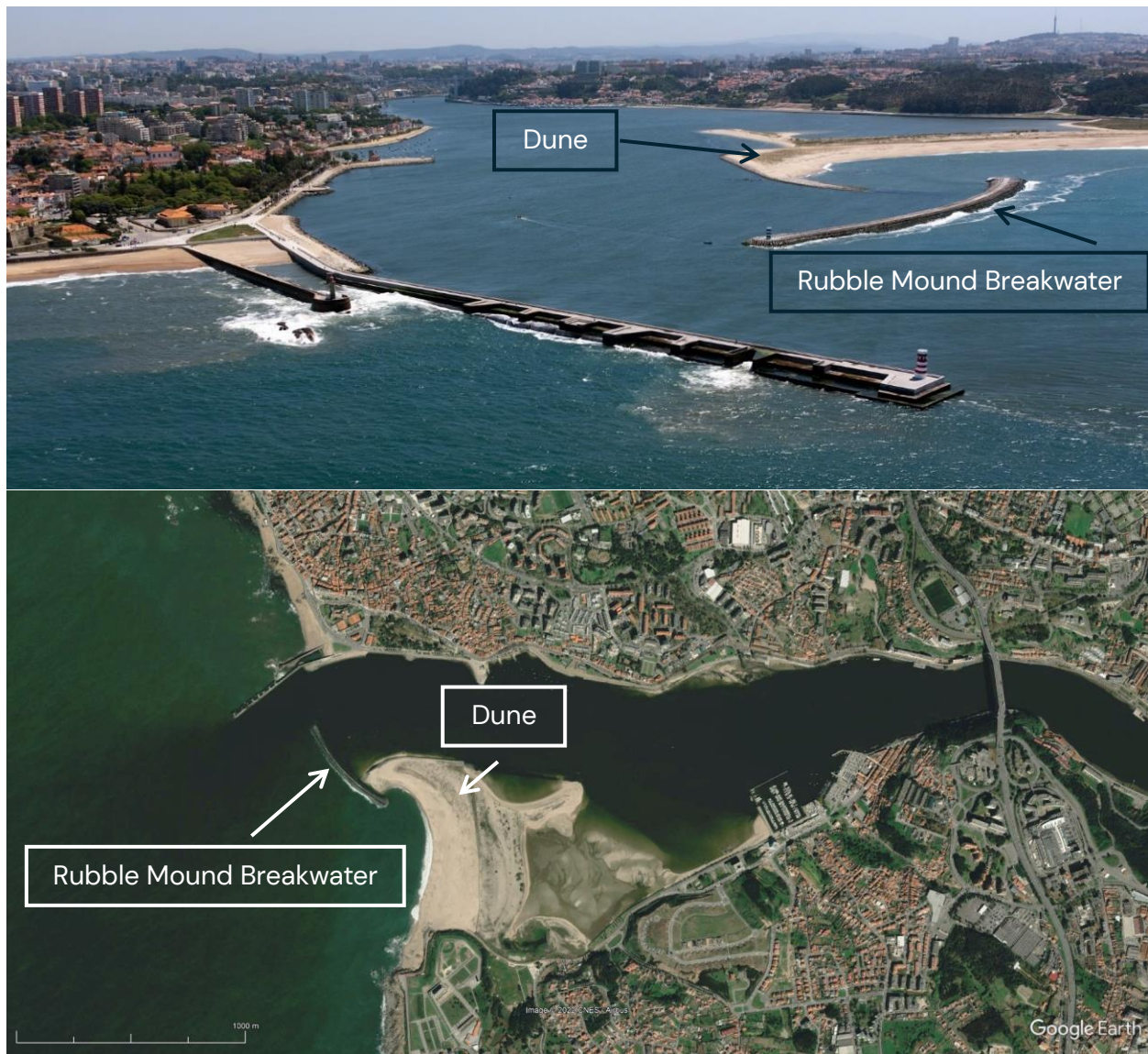
Figure 4 – Douro estuary sandspit (PT) Demonstrator, a rubble mound breakwater in front of a Dune
