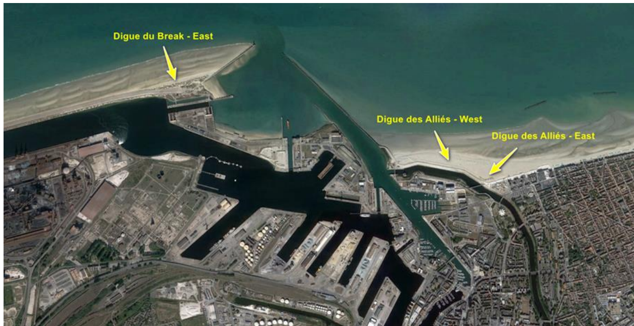
Figure 6 – Dunkerque (FR) Demonstrator, at three key locations: Malo les Bains (West and East sections of the Digue des Alliés) and Digue du Break
