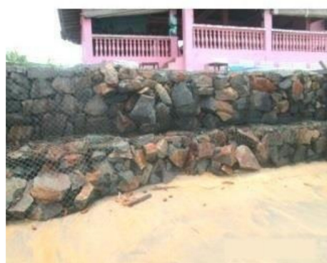
Construction of a protective stone bund in Mboamanga
