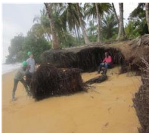
Protection of the banks against marine erosion
