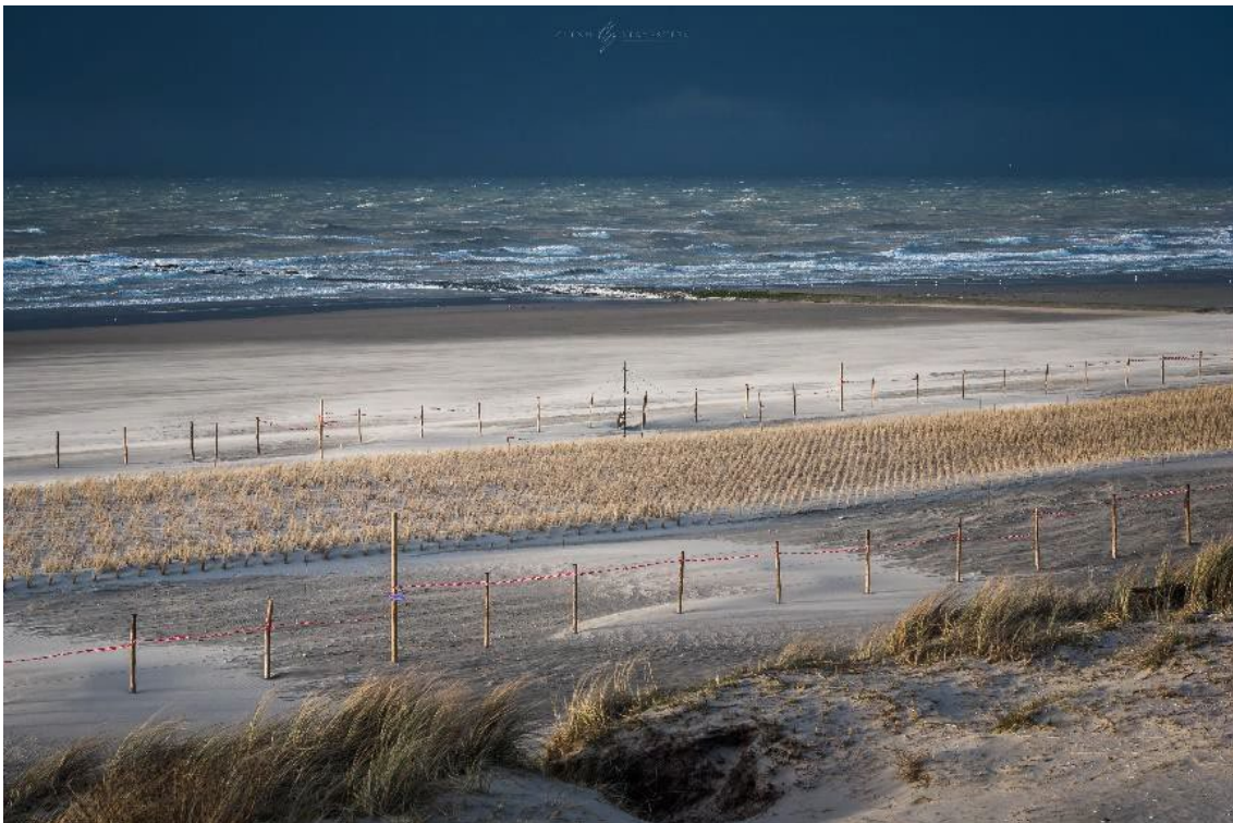
Figure 1: Location of the dune-in-front-of-a-dike in Oosteroever, Belgium (image taken on 11 March 2021). Within the engineered dune design marram grass is planted in different spatial distributions with three densities. The dune is surrounded by a fence to prevent beach passage.
