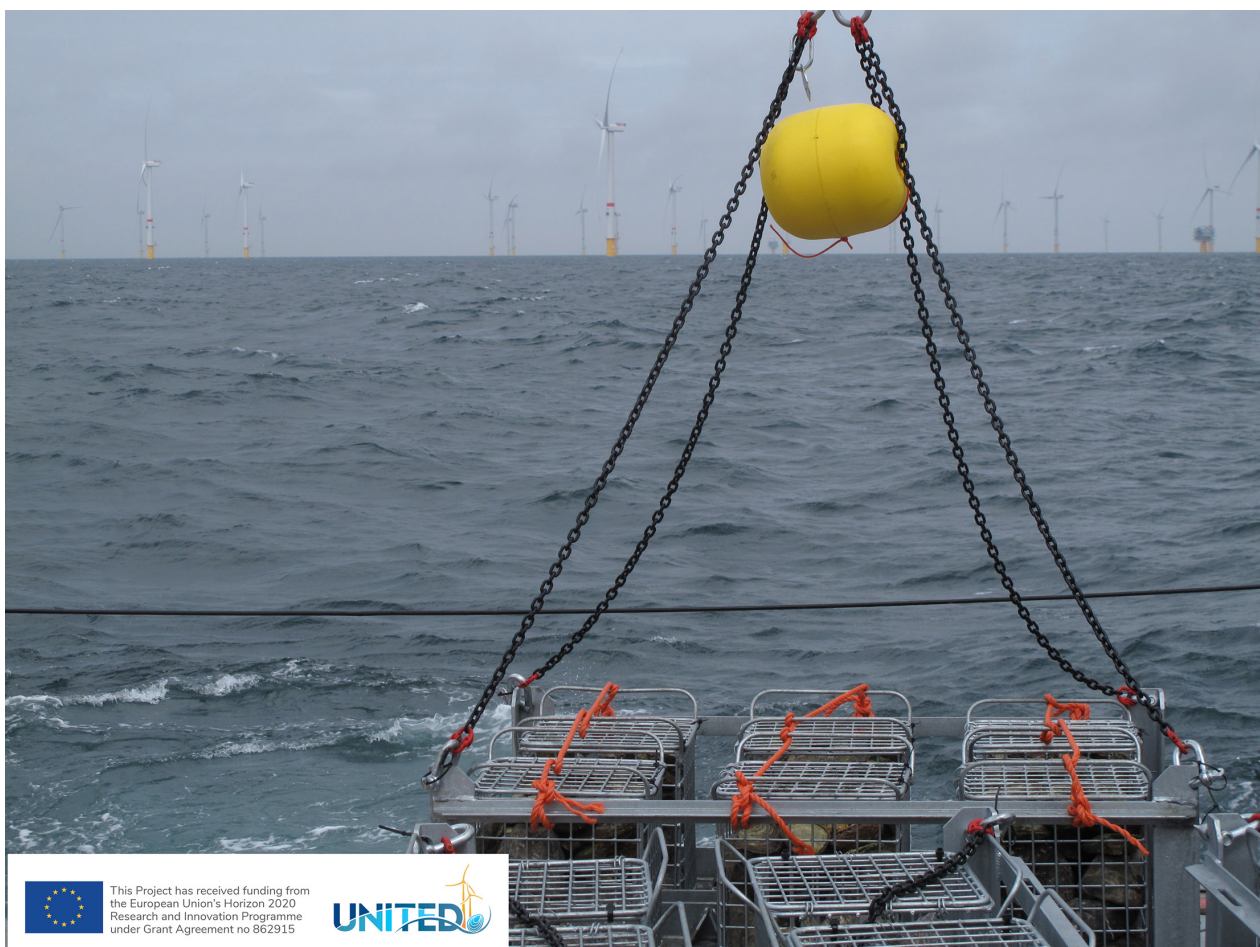
Figure 4. Installation of ‘oyster tables’ to facilitate restoration of European flat oyster ( Ostrea edulis ) reefs in the Belwind wind farm as part of the EU Horizon 2020 project UNITED (© Annelies M. Declercq).
