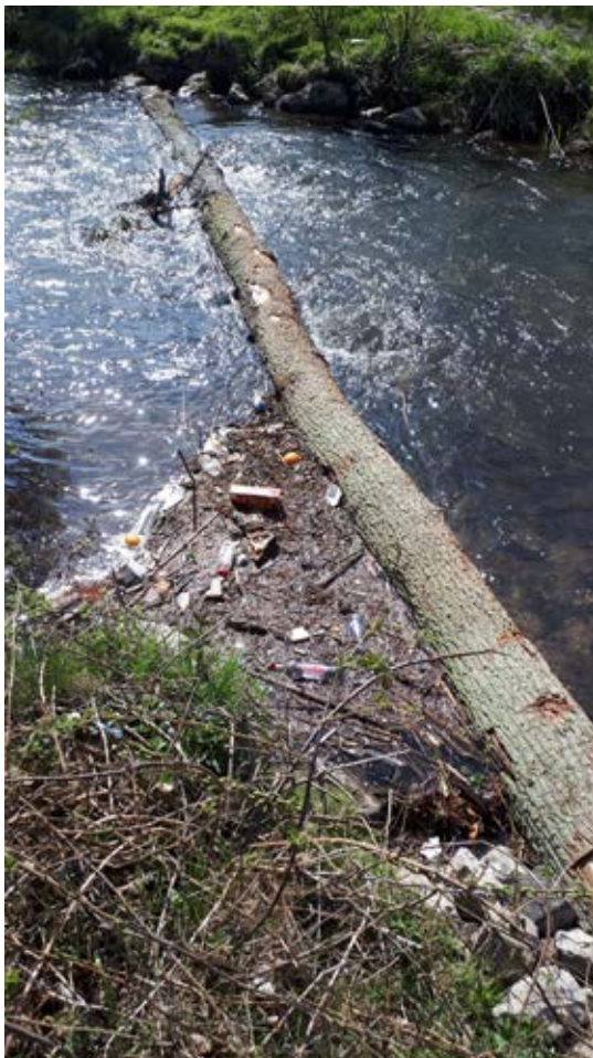
Float beam placed by WVER
