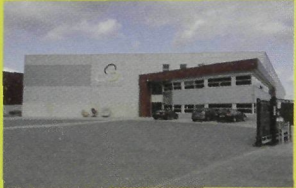
New foundry and office
