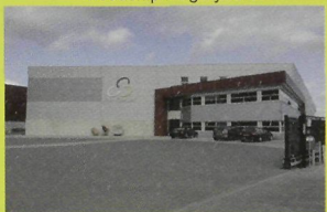
New foundry and office
