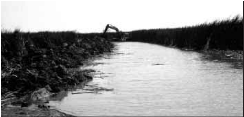
Picture 9: In 1998, clearing operations were carried out by an amphibious mechanical digger.
