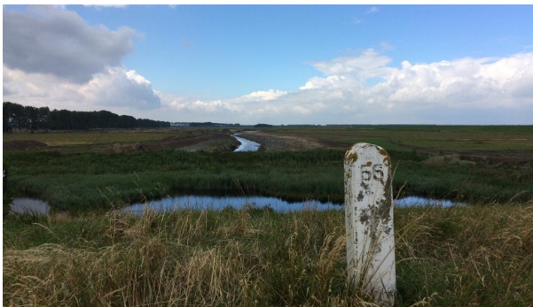
Figure 1 Excavated creek inside the polder. Photo taken from the Scheldt dike looking towards the polder. The Sieperda dike is visible in the far right. Photo by K. van den Hoven.
