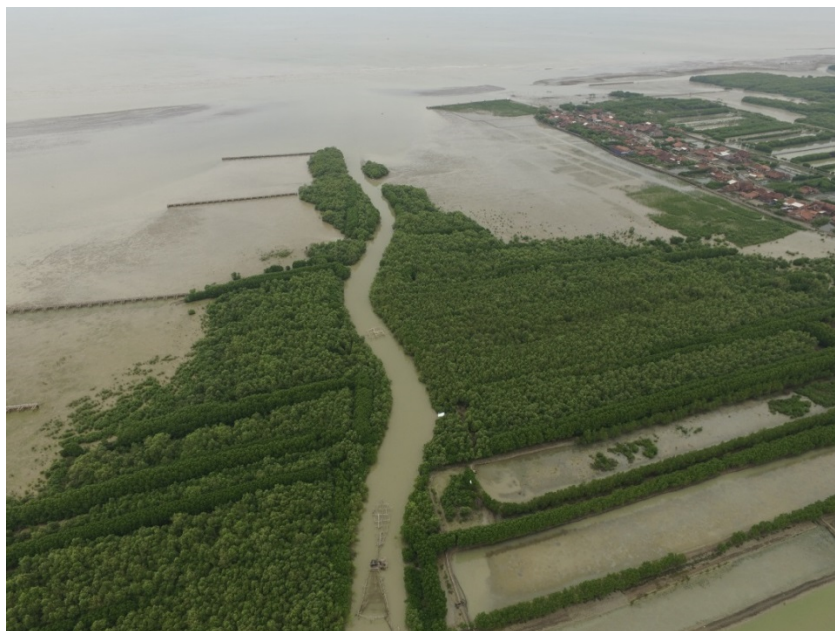
Drone image of the project location in the coastal zone of Demak district in Indonesia. The dams on the left attenuate incoming waves, stimulating the deposition of sediment to ultimately encourage mangrove re-establishment.
