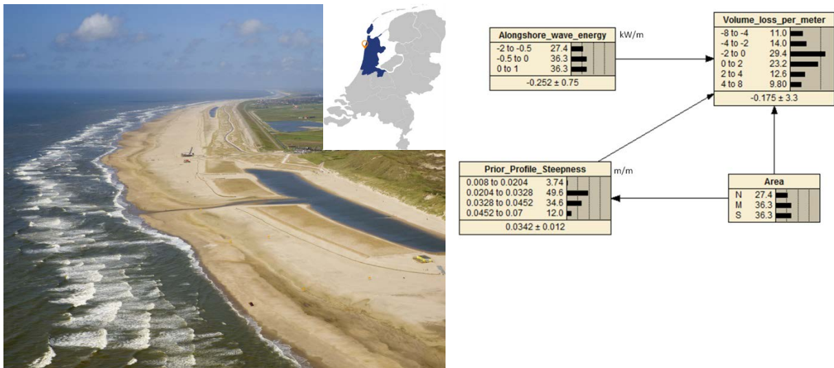
Left an aerial picture of the HBD just after installation. Right: The Bayesian Network with first year of observations.
