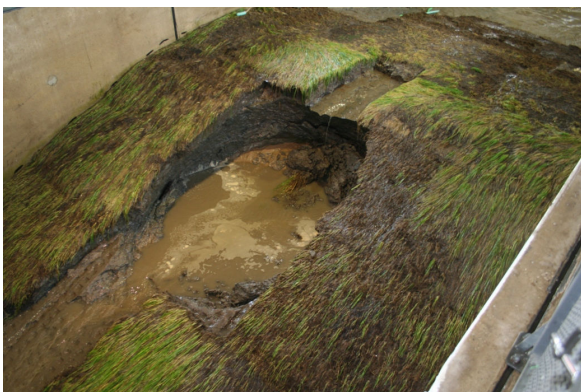
Fig 2. Breach development caused by overtopping
