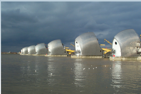
Fig. 1. Thames Barrier - part of the flood defence system in the Thames estuary
