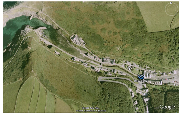
Fig. 4. View of flooding location - Boscastle
