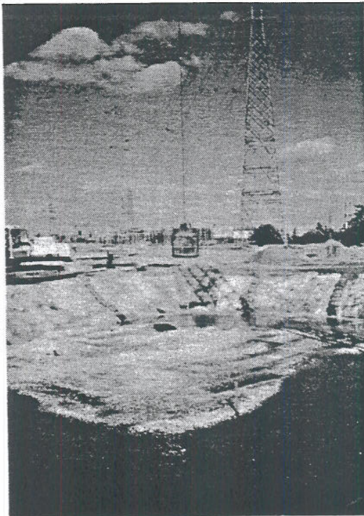
Picture 3 : Testing weight ready for impact test
