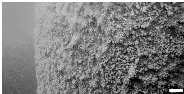
Fig. 3 Freeze-frame from the underwater video of the B8 monopile (for location, see Fig. 2) at the Belwind I OWF on 2nd June 2010, 7 months after piling. Bio-fouling is mainly by the hydroid Tubularia larynx (F. Kerckhof, pers. comm.). In the water column, marine snow or fine-grained flocs are visible. Scale bar 15 cm. Photograph taken by A. Norro, RBINS-OD Nature
