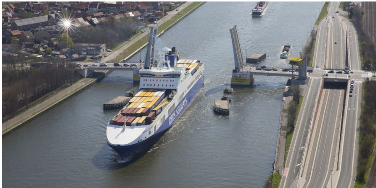
Figure 52. Bridge on the channel Ghent-Terneuzen at Zelzate [111].
