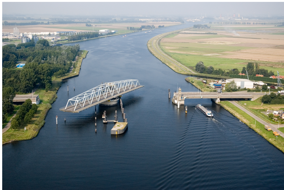
Figure 37. Turning bridge on the channel Ghent-Terneuzen at Sas van Gent [97].
