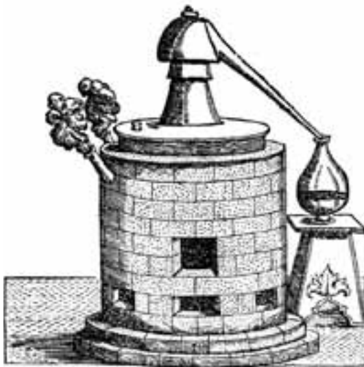
Fig. 35: Equipment for the distillation of Amber, from Mattioli (1565).
