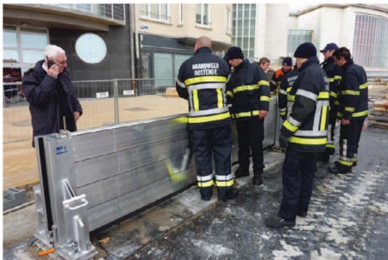
Figure 4: Firemen setting up the mobile storm wall.
