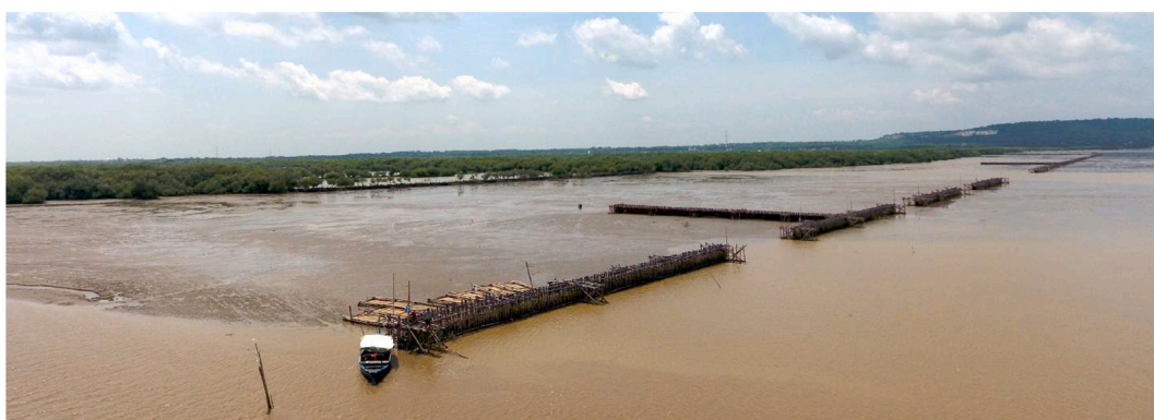
Fig. 8. Example of permeable dams in Gresik Regency, close to Solo River, Java, Indonesia (photo by MMAF early 2019).
