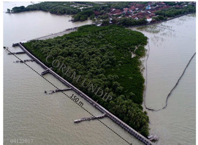
Fig. 9. APO, concrete seawall at Timbul Sloko, Demak, Indonesia (courtesy COREM-UNDIP) with natural colonization by Avicennia (high vegetation) and planted Rhizophora (low vegetation).
