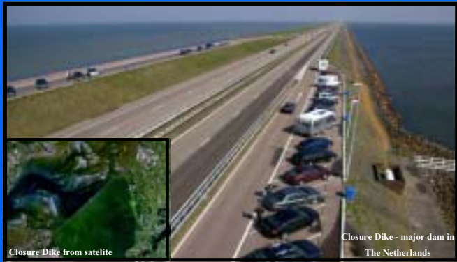
Closure Dike from satellite
