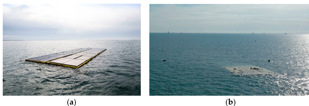
Figure 1. (a) First two modules of the offshore floating solar array of Oceans of Energy installed nearshore in the Dutch North Sea in 2019; (b) Sixty-four (64) interconnected modules creating a floating farm with one-third the size of a football field, operational 12 km offshore from The Hague, the Netherlands since 2020. Farm will be expanded to 1 MW-size in 2023; 1 MW-size is approximately one football field large [7].
