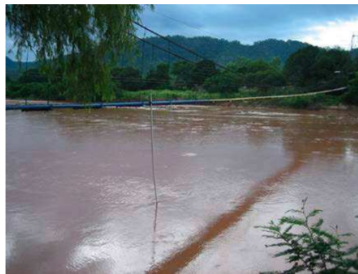
Figure : Installation of the limnimeter in the Rio Parapeti. The pressure probe is inserted into the pole.
