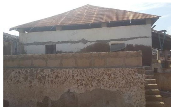
Extension of the outer wall of the water tank in progress
