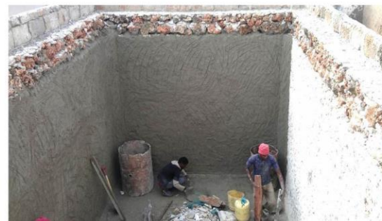
Construction work on the new water holding tank in progress
