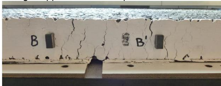
Figure 3: Specimen after cracking in joint-tester at Breijn-Heijmans.
