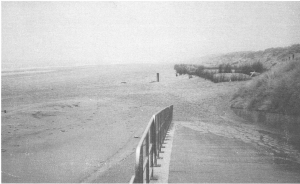
Figure 2. Beach at De Haan after nourishment and placement of berm (Belgium) (Photo: Haecon, nv).
