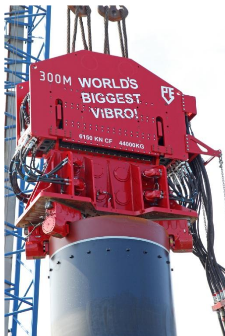
Figure 37. PVE 300M Vibratory hammer clamped directly to a monopile. (Starre & Boor, 2011)
