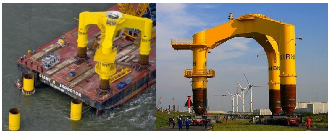
Figure 53. Tripile foundation used by BARD GmbH for its offshore wind parks (© BARD Engineering GmbH)
