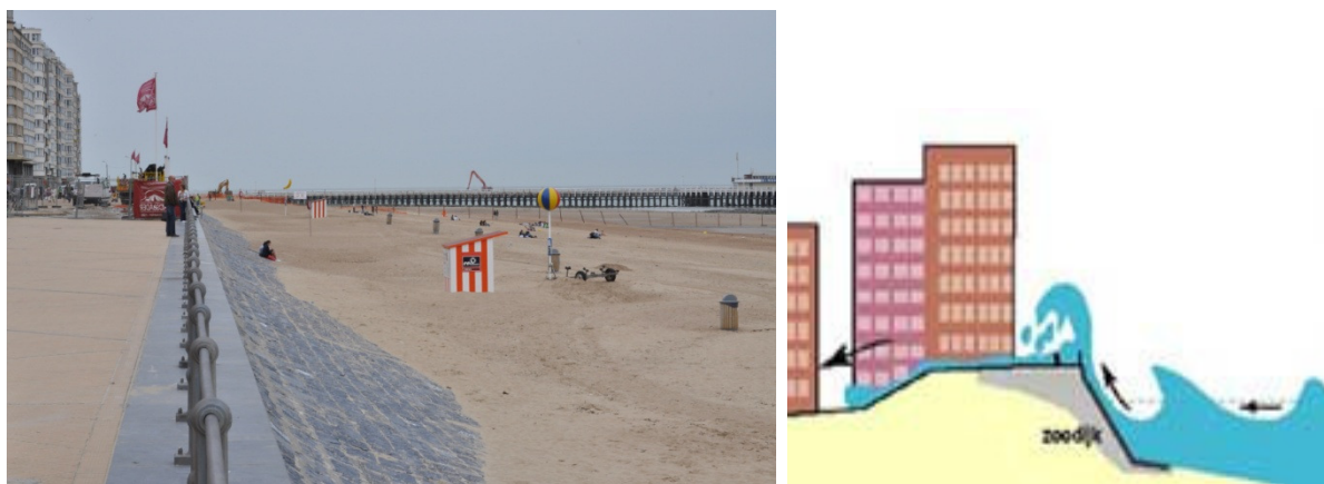
Figure 1. Typical dike geometry along the Belgian coast (left), causing dangerous situations during a storm (right)
